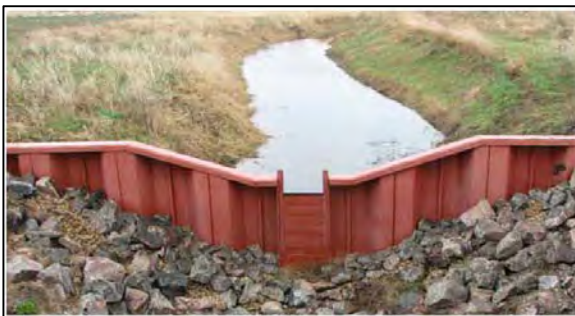
FIGURE 21 EXAMPLE WEIR WITH STOP LOGS TO ADJUST WATER LEVEL
