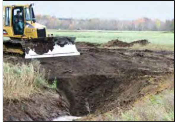
FIGURE 19 EXAMPLE OF AN EARTHEN LATERAL DITCH PLUG INSTALLATION
